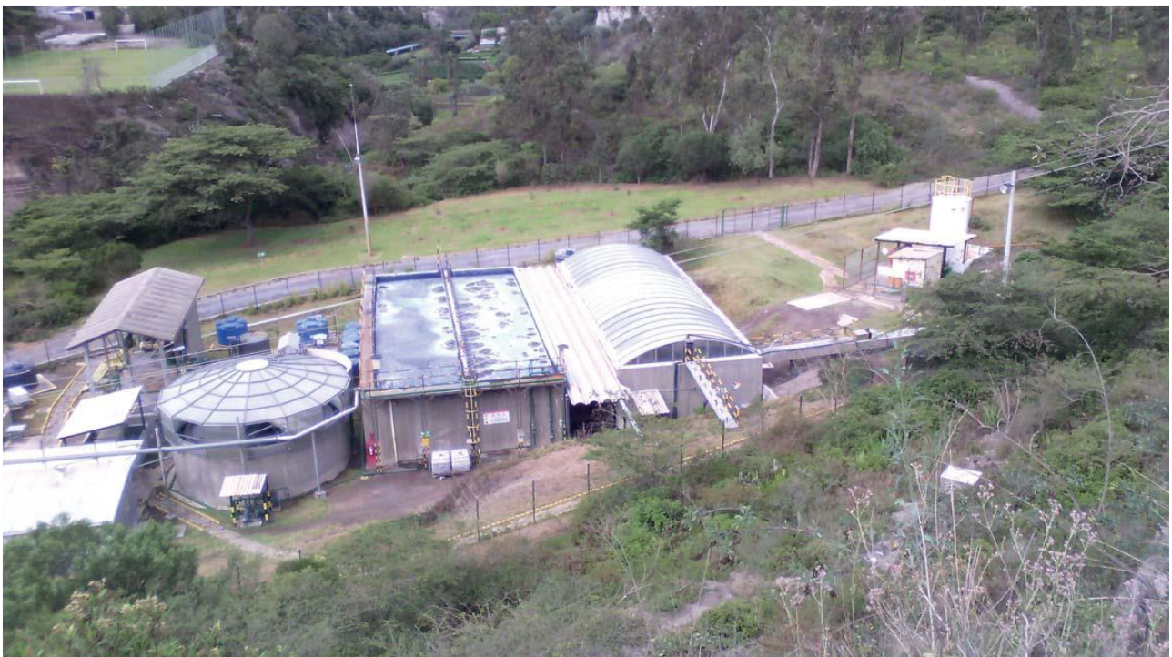
AFTER: 100% Biological treatment Plant by IDROSISTEM
