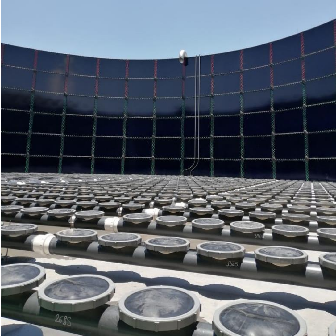
AIR DIFFUSERS INSTALLED AT THE BOTTOM OF THE BIOLOGICAL OXIDATION TANK
