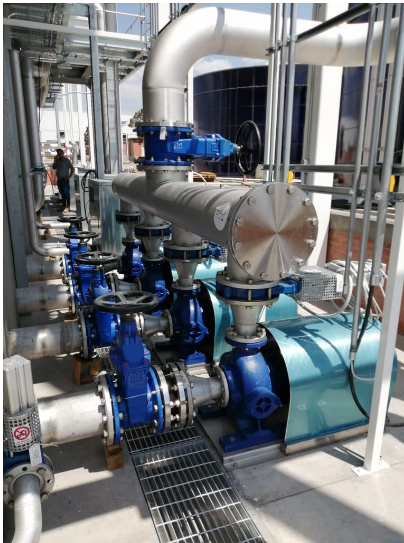
CENTRIFUGAL PUMPS FOR SLUDGE RECIRCULATION IN YAZBEK
