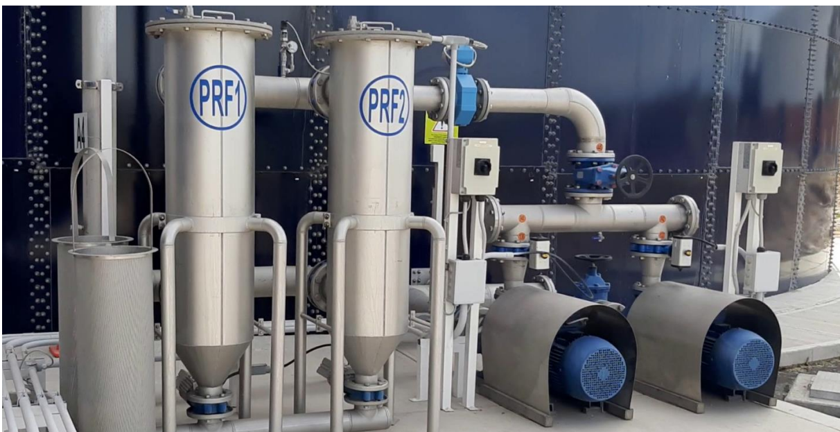
PRE-FILTERS PLACED BEFORE THE BIOLOGICAL OXIDATION TANK
