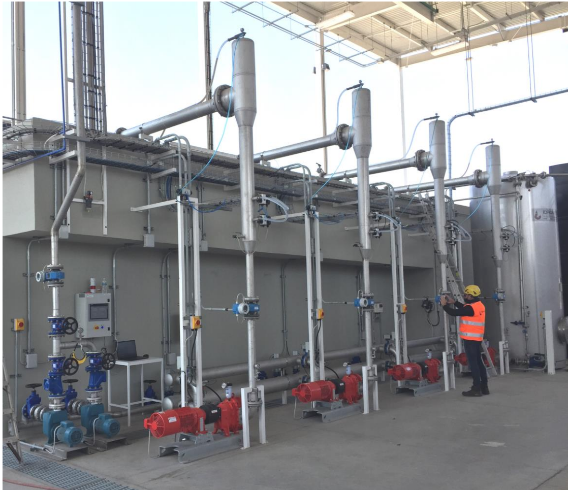
MBR MODULE WITH ULTRAFILTRATION MEMBRANE
